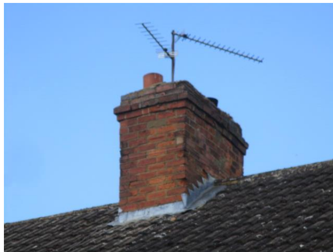
Repairs to chimney.
