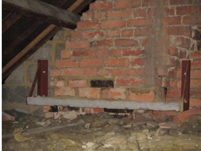
Support for removed chimney.
