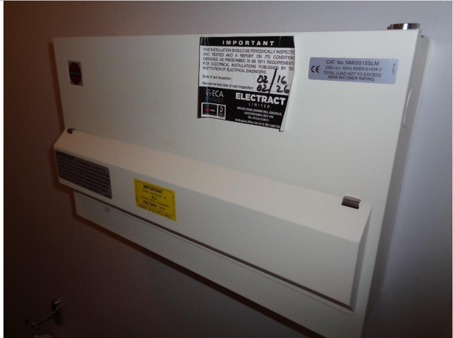
RCD in cloakroom Condition Rating 3.
