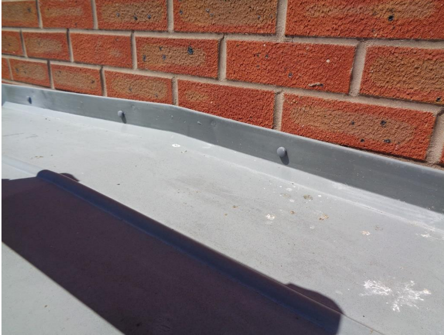
Fibreglass covering to front canopy
