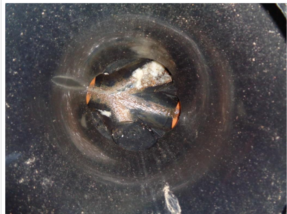
Rear drain to right needs flushing through
