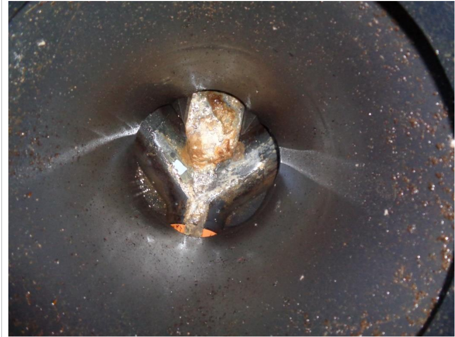
Front drain to right needs flushing through
