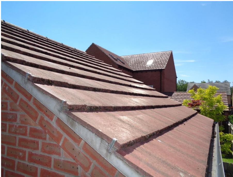
Rear roof slope of garage
