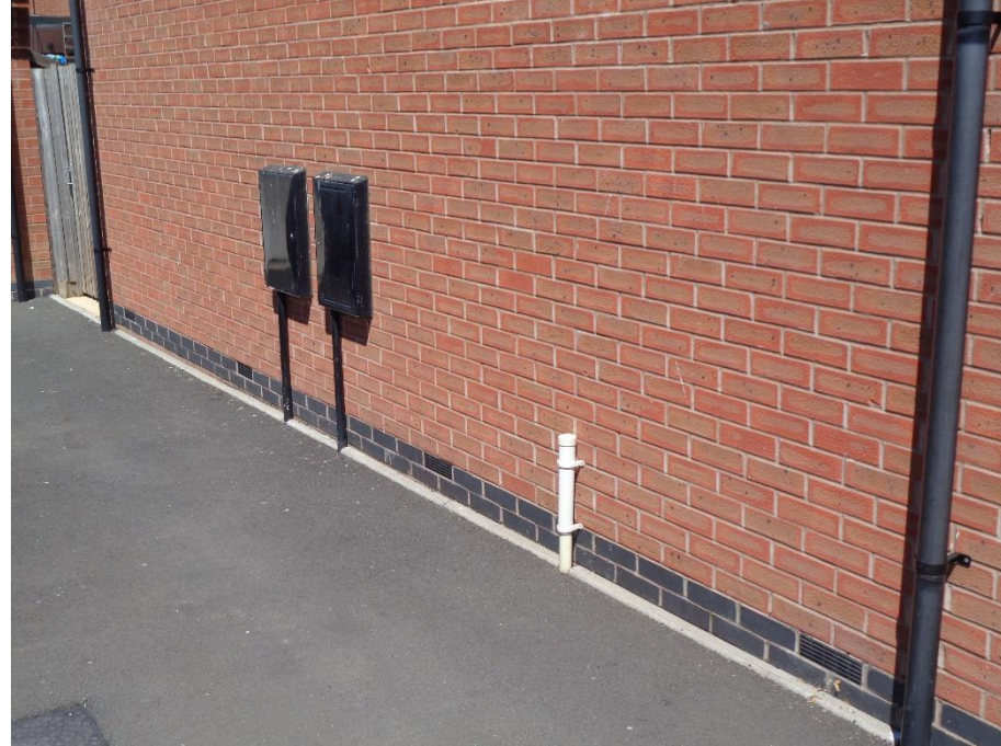
Ventilation to suspended concrete flooring Condition Rating 1.
