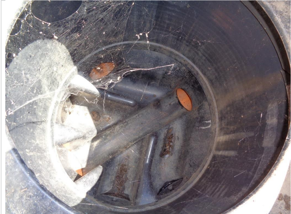
Drain to driveway running clear
