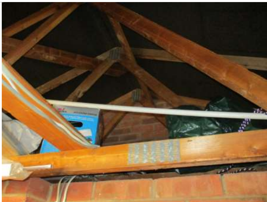
Garage roof structure
