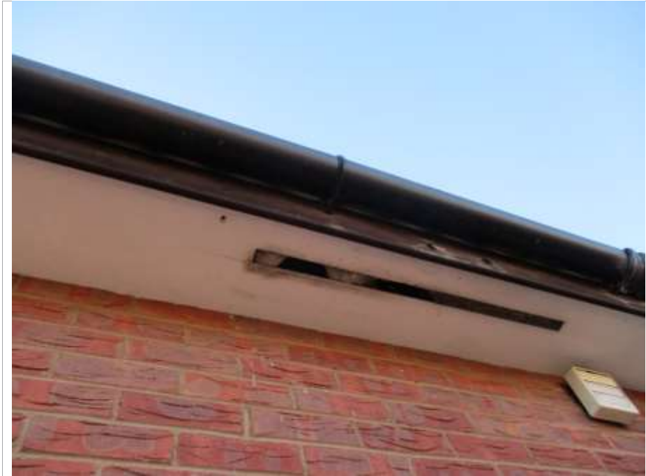
Ventilated cement asbestos soffit boards Condition Rating 2
