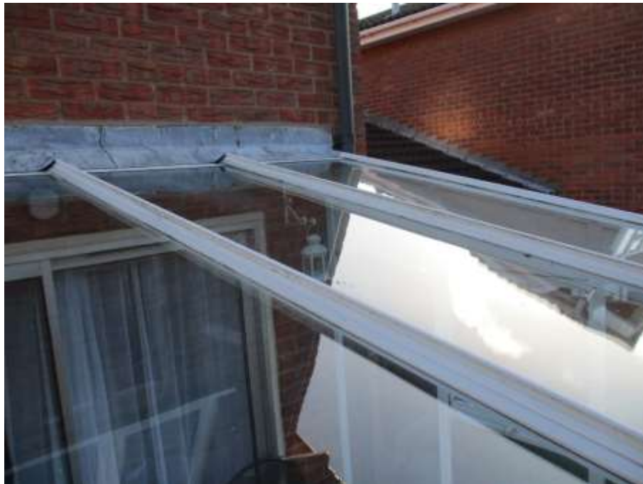
Lead flashings to conservatory roof
