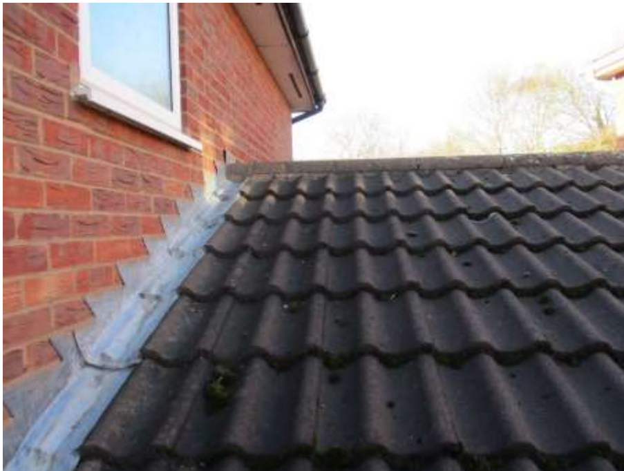
Lead flashings between garage and main wall
