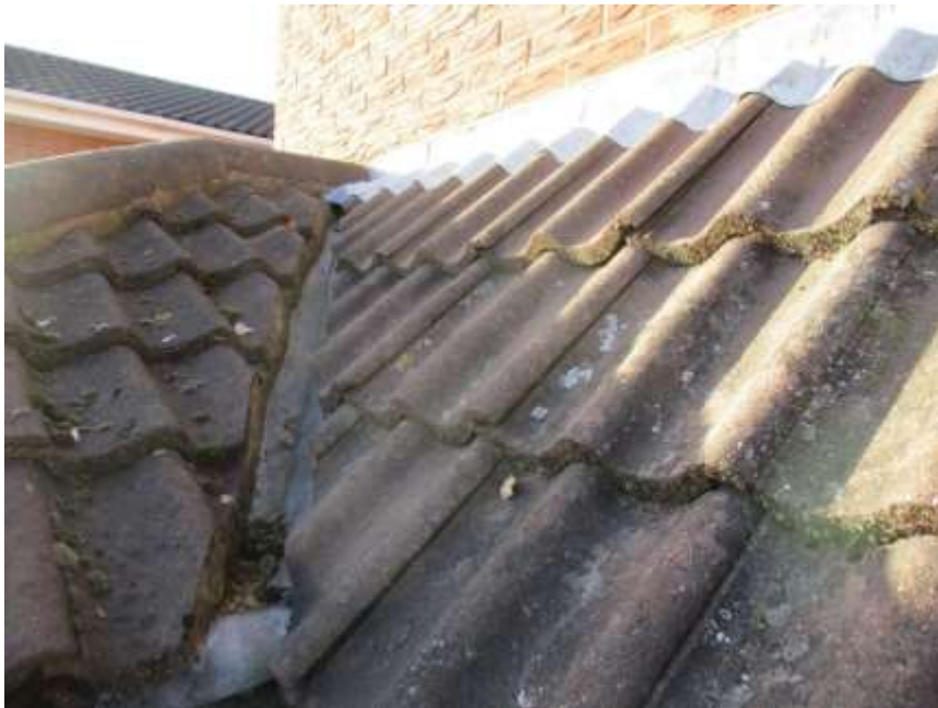
Valley to porch clear
