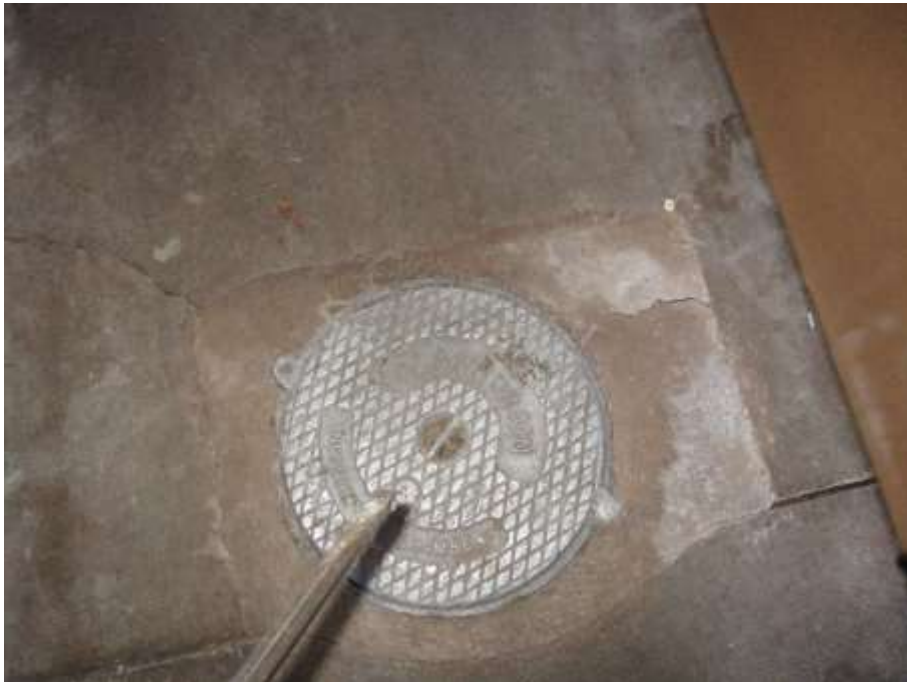
Screw sealed down to rodding point
