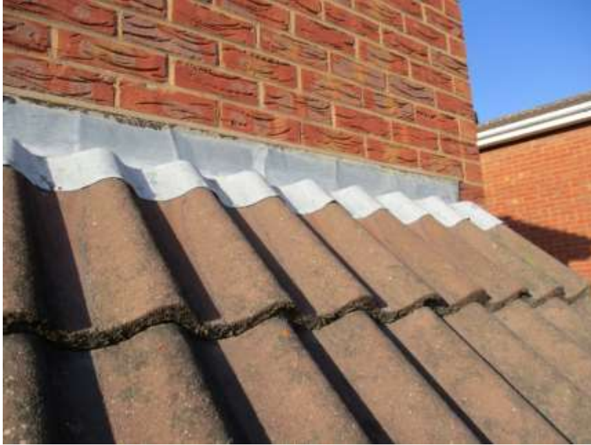
Lead flashings satisfactory
